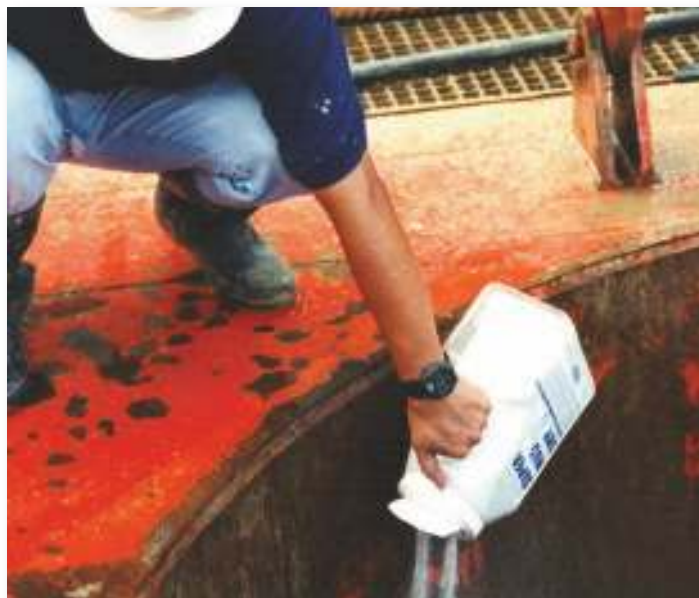
Mixing Directly into the Excavation
